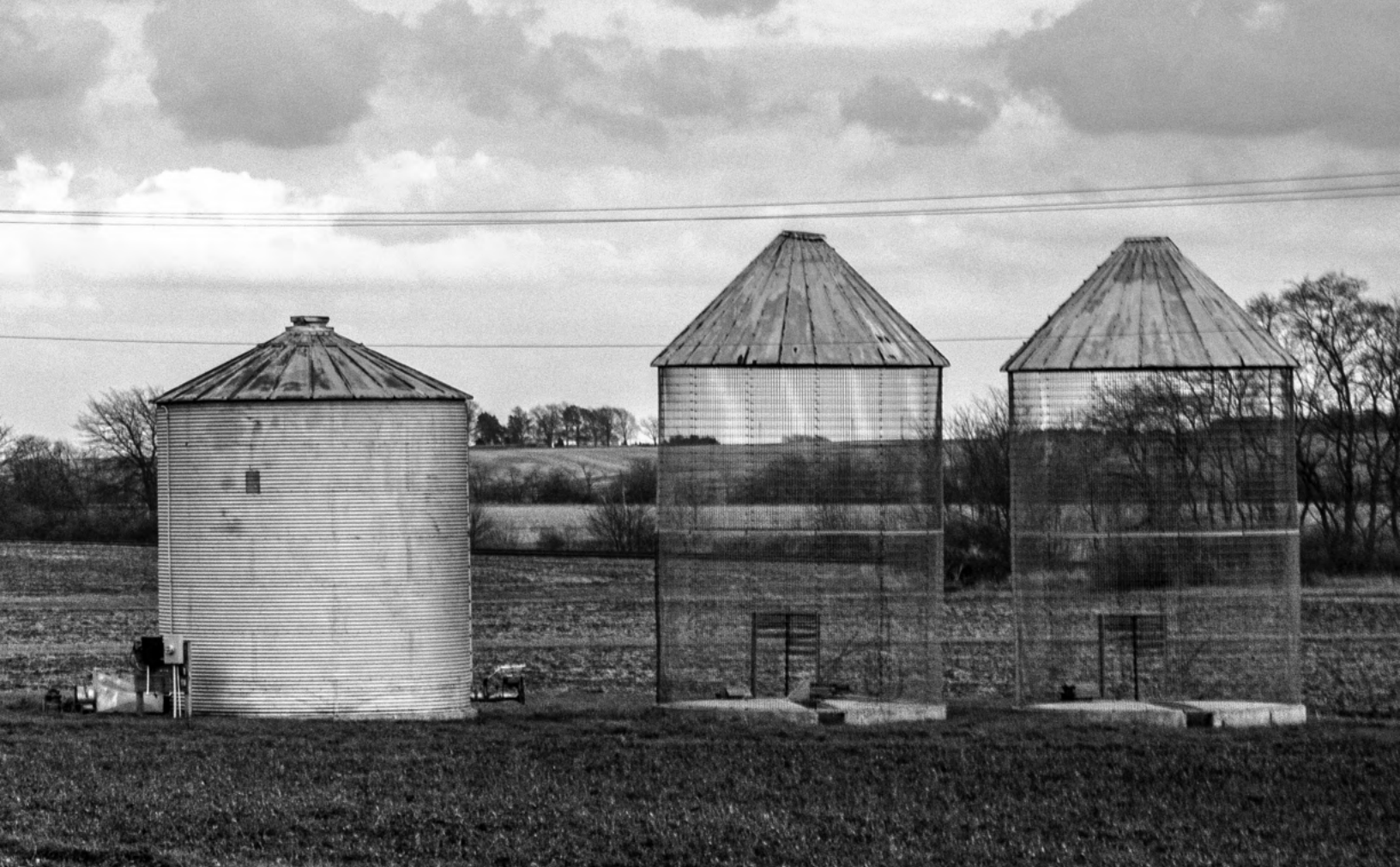
Grain and Corn Silos - Central Illinois
